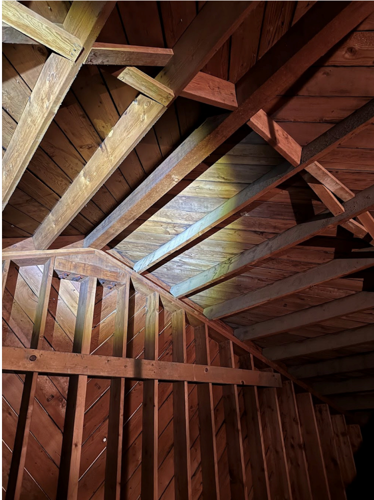
Figure 1. Attic View of Wall and Roof Diagonal Sheathing.
